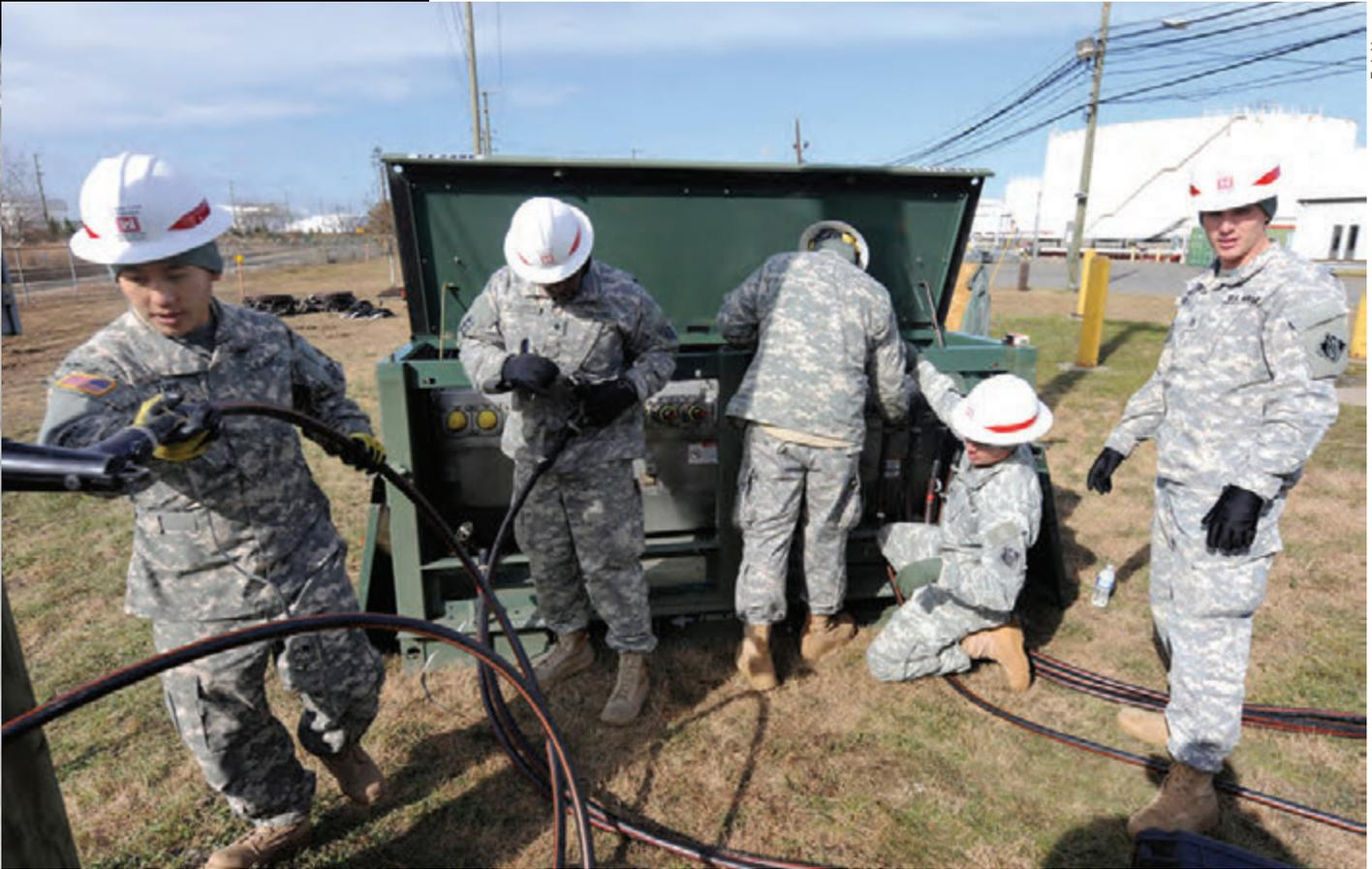
Soldiers install electrical generator equipment at a Carteret, N.J., fuel depot that lost power during Hurricane Sandy. DLA Energy provided fuel to state, local and federal responders for electric generators and water pumps.
